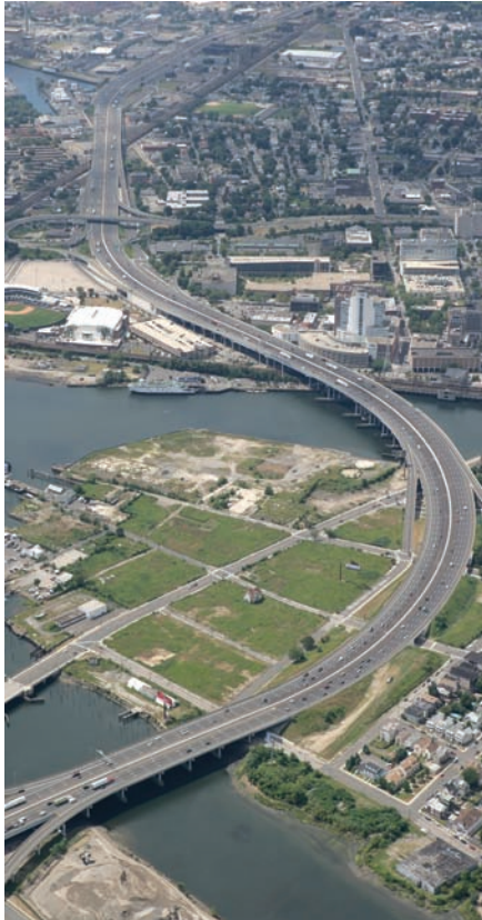
Connecticut is spending $200 million of the $1.6 billion it received on highway and bridge repair, including stretches of the state's major thruway, I-95.
