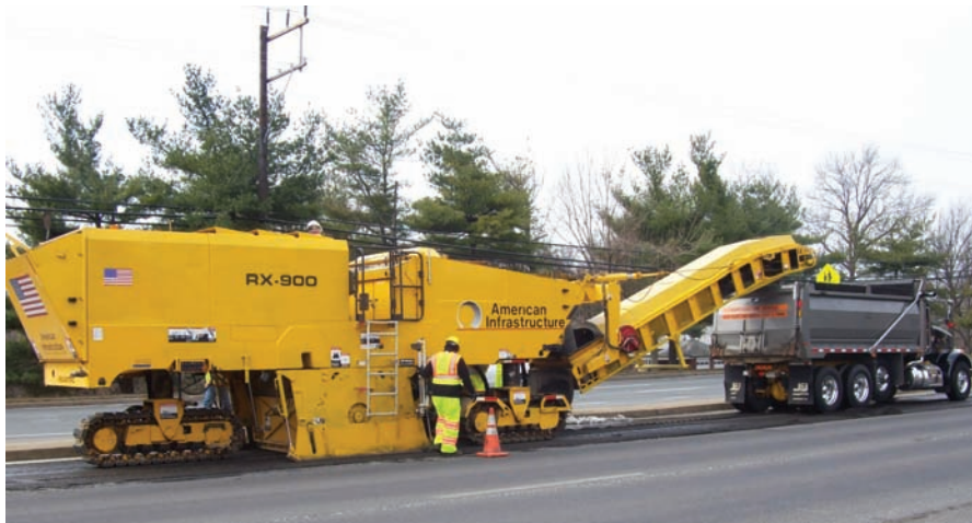
On March 4, Maryland awarded a $2.1-million road resurfacing and improvement project along New Hampshire Avenue in Montgomery County to American Infrastructure. (Photo courtesy American Infrastructure)
